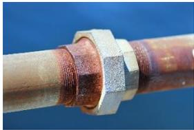
Follow all water tubes, pipes and connections looking for leaks.
